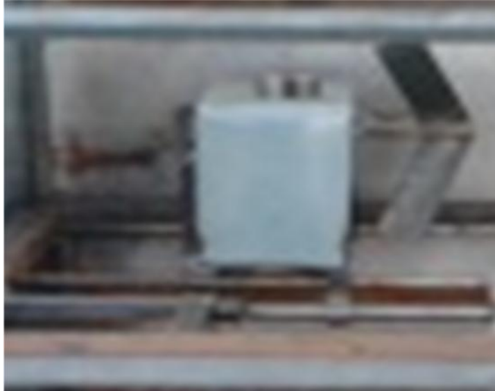
Gambar 3.33. Pemasangan housing penjepit
