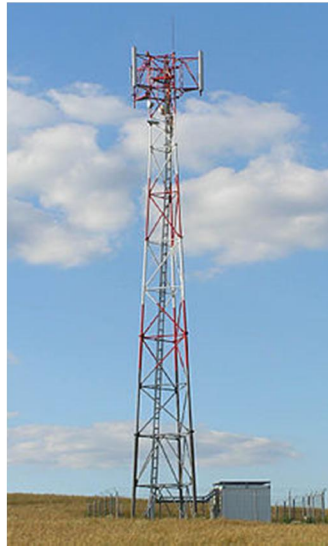
Gambar 2.15 - Menara BTS (Based Transceiver Station) 34
