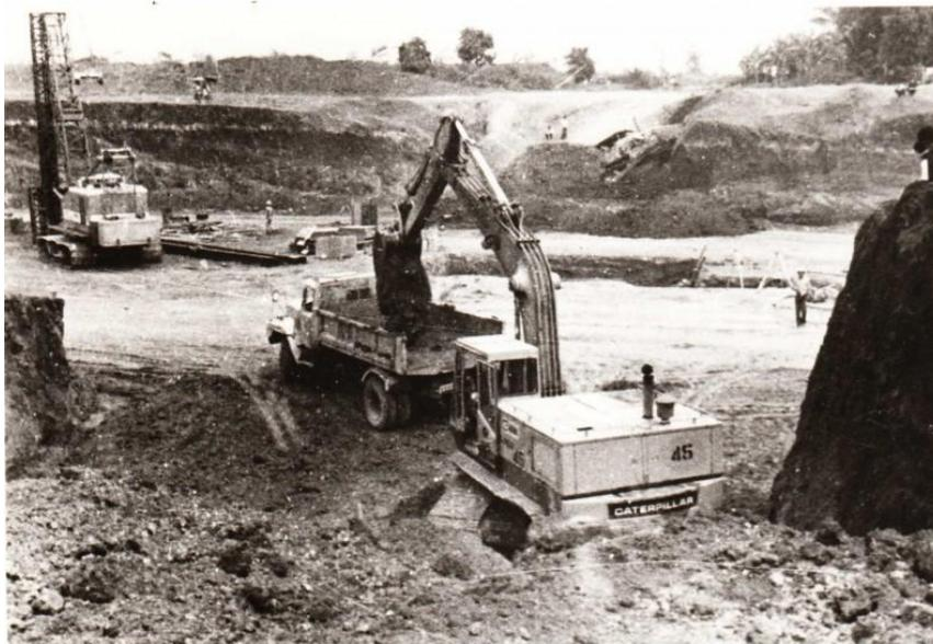
Roadway excavation using loader and trucks
