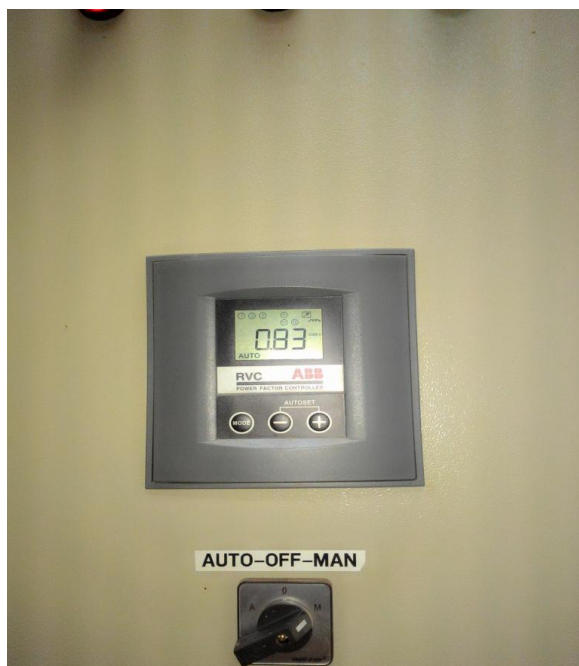
Gambar : Pengukuran Faktor Daya di Power Factor Regulator Saat Capasitor Bank
