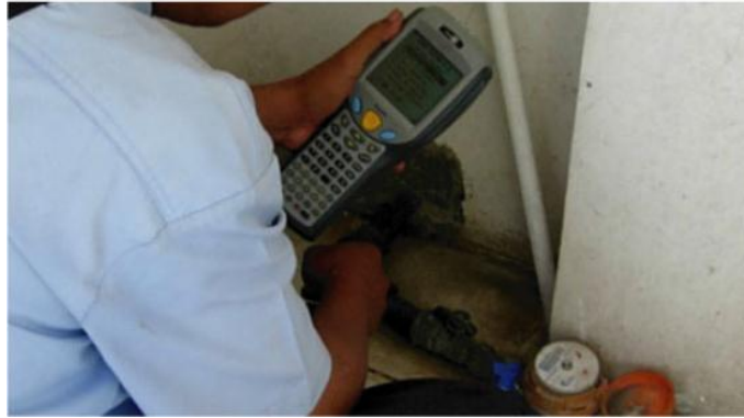
Gambar 2. 3 Proses pencatatan meter air (AETRA, 2015)
