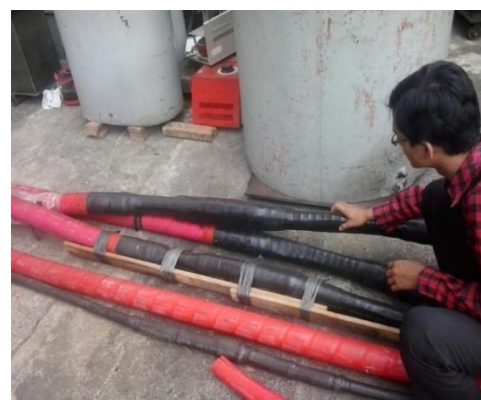
Gambar 2.7 contoh kabel jointing
