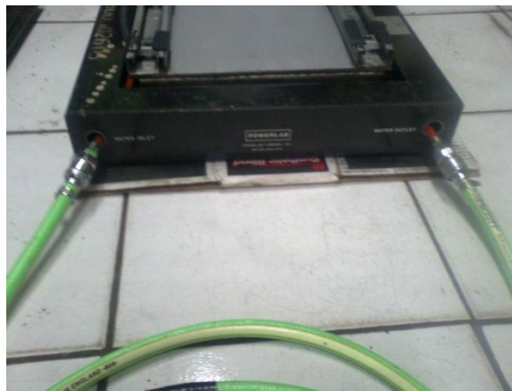
Gambar 3.11 Pemasangan Water Hose
