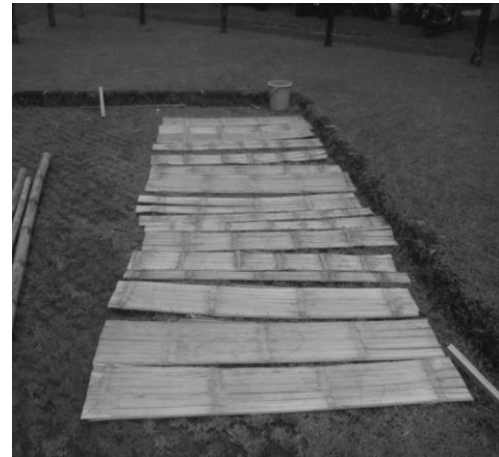
Gambar 3.16 Proses penjemuran palupuh
