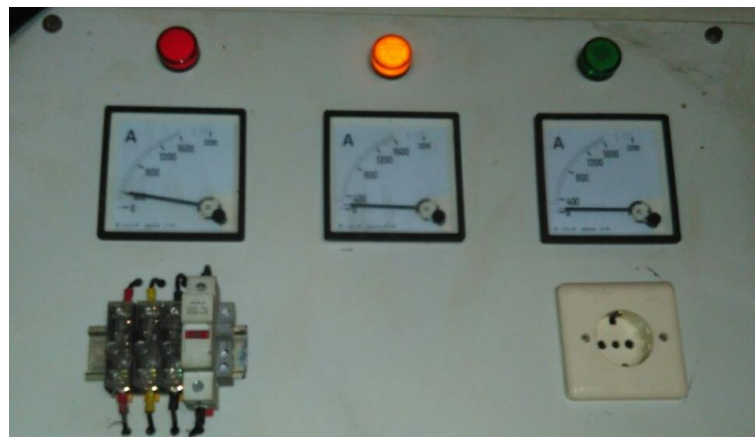
Gambar 2.7 Sirkit Bantu PHB TR
