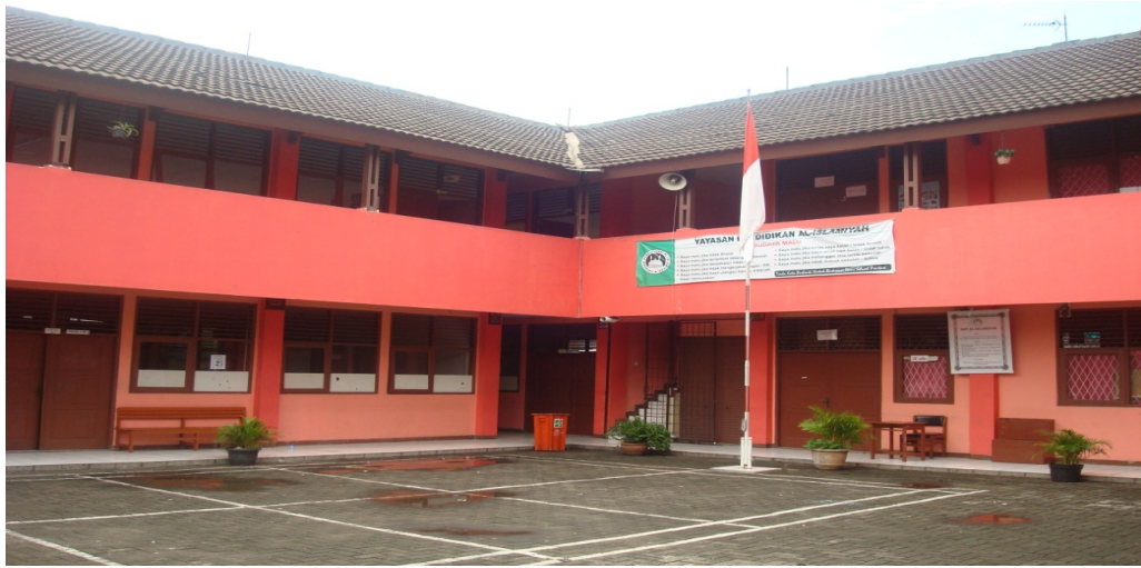
The school looked from front side
