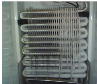
Gambar 2.21. Frosting Evaporator 34
