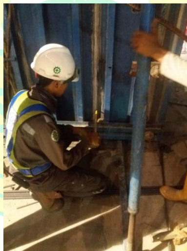
Gambar 4.16 Cek Vertikality Bekisting Kolom
