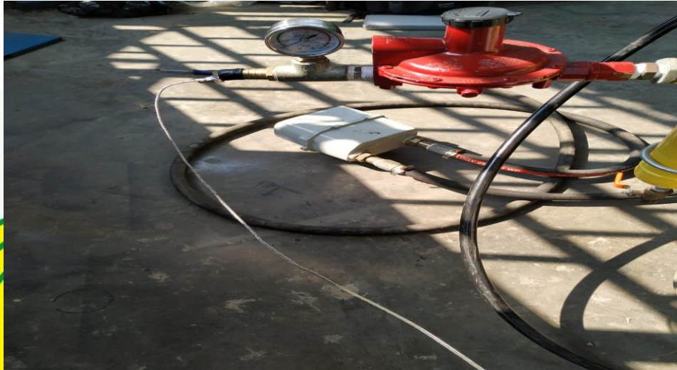
Gambar 3.9 Pengujian temperatur gas di regulator
