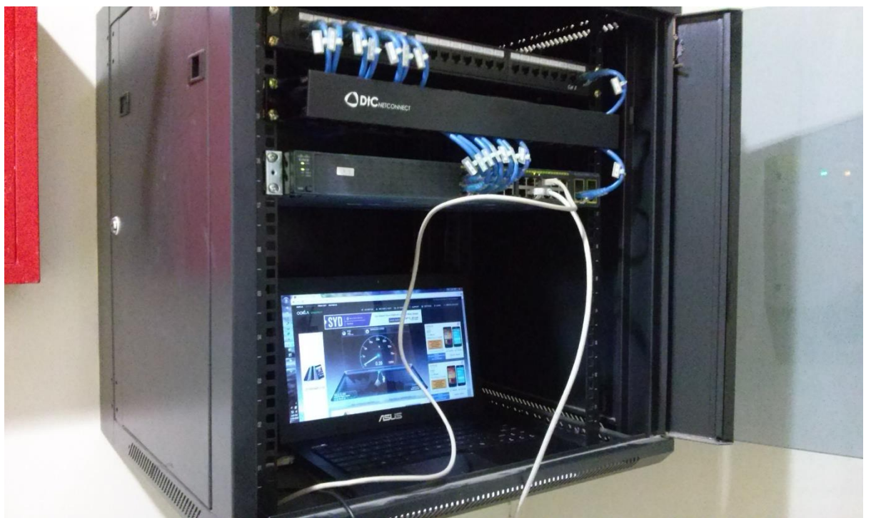
Switch Cisco Catalyst 2960 Lantai 2 – Lantai 10
