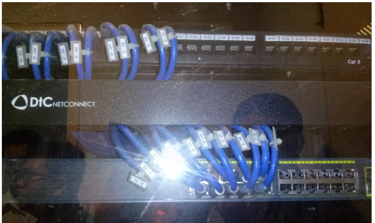
Switch Cisco Catalyst 2960 Lantai 2 – Lantai 10
