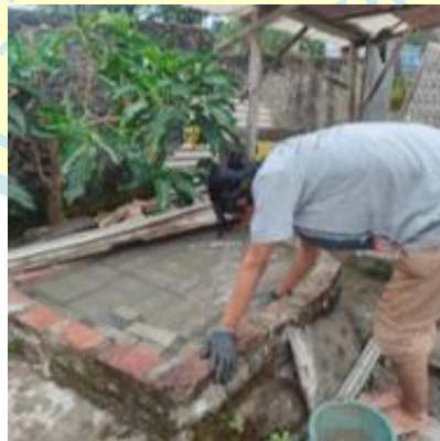
Gambar 4.6 Proses Perawatan Paving Block
